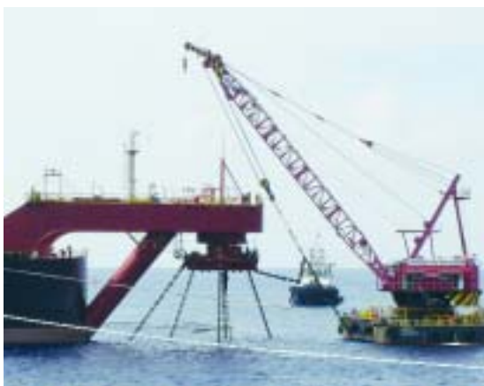
Our crane barge, Isamigo 3, handles the on-location chain replacement
