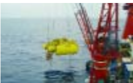
Mid Water Arch (MWA) installation
